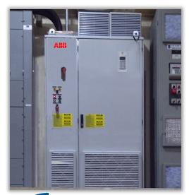
The ACS800-37LC drive installed on the mezzanine at the City of Lawrence pump station
