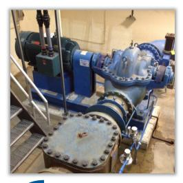
The Baldor 350HP motor installed next to City of Lawrence's pump #4
